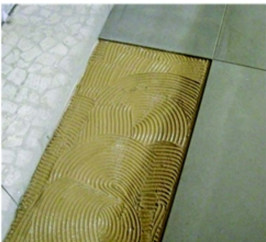
Floor panels set using elastic polyurethane mortar
